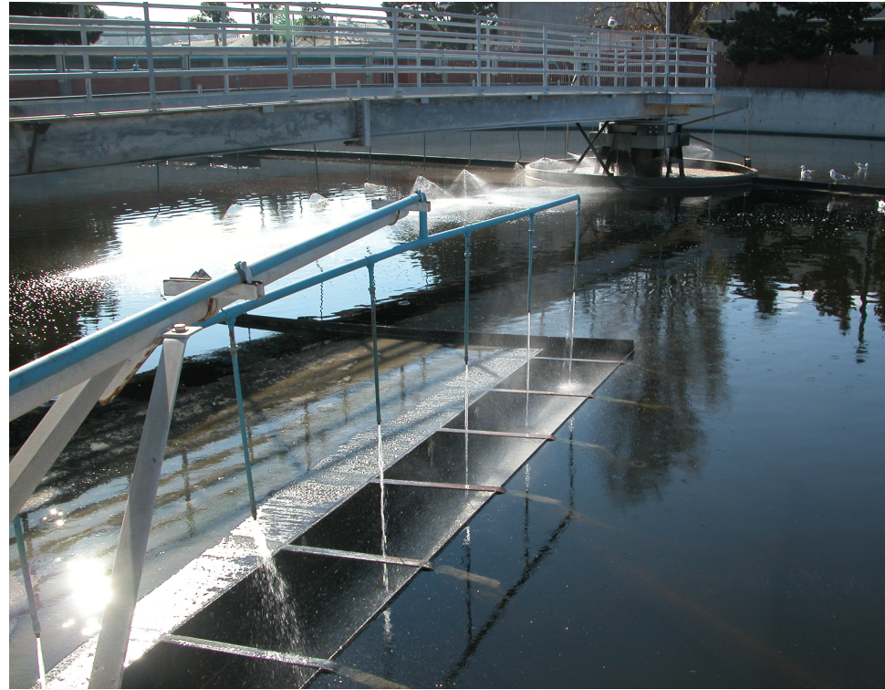
Clarifier at Southeast Treatment Plant
